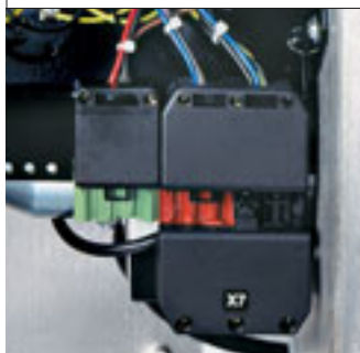
Example of the terminal board for electrical connections on RL 28 - 38 burners
