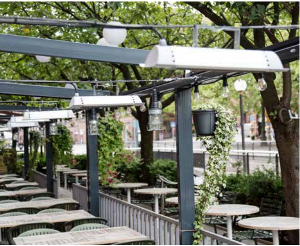
Thanks to a high temperature of 2200 °C and the adapted reflector, IH is extremely efficient and provides a comfortable heat.
